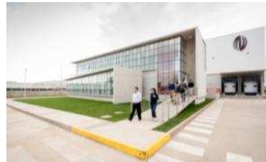
Factory in Santiago, Chile operational
